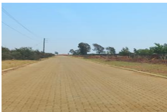
Block paved road
