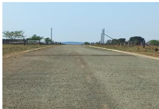
Double Sealed road
